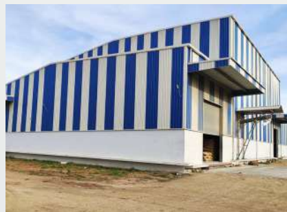
Mr. Balaji, Pre Engineered Building
