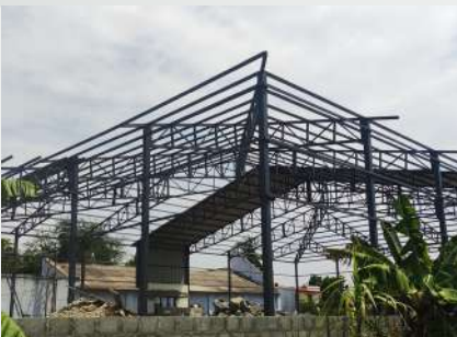
Mr. Dhanabal, Roof Truss
